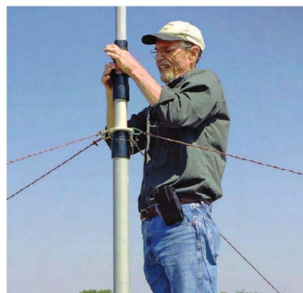
Figure 6 — Dayle Good, KK6HNS, pushing up mast sections while helpers gently hold the top guy wires.
