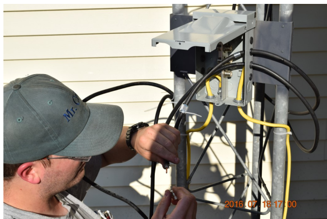
Joe had already pulled the cables from his shack. Peter finished work by terminating the cables.
