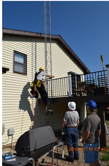
Peter KB(WZD) starts up the tower. The antenna stayed on the ground until he was ready. At that point Lloyd Vandervoort N9RPU attached it to a rope and Peter pulled it up.
