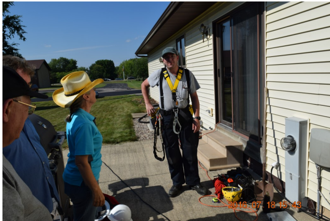
Peter Fox KB9WZD finishes preparation before climbing the tower to install the two antenna's Note the safety gear and the even more elaborate than
